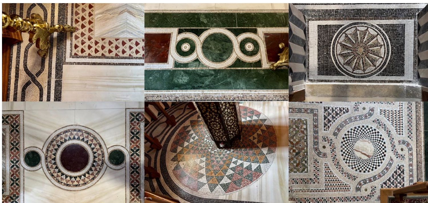
Close-up details of the intricate patterning of the new hand-laid marble floor in the katholikon, Pantokratoros Monastery
