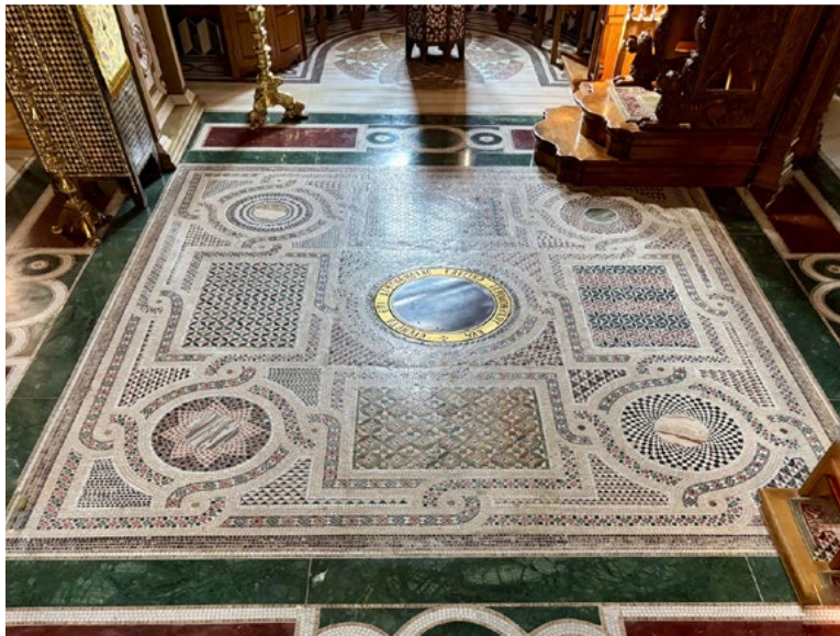
The new hand-laid marble floor in the nave (naos) of the katholikon, Pantokratoros Monastery
